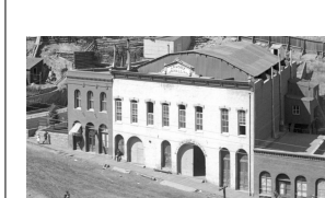
3 EAST ELEVATION HISTORIC PHOTO NTS
